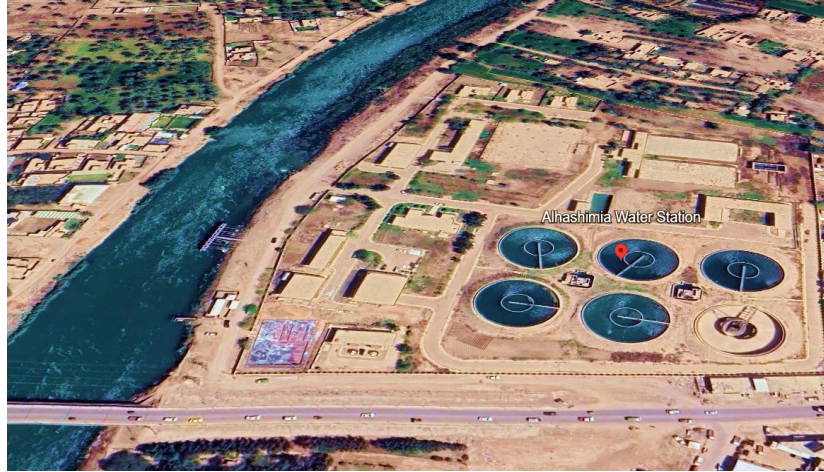
Figure 1: Al-Hashimiyah water treatment plant (Google Earth)
